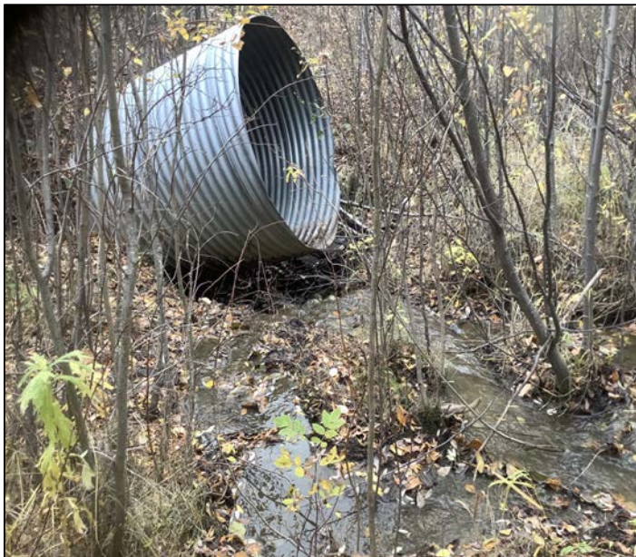
Photo 1. Facing right downstream bank towards inlet
