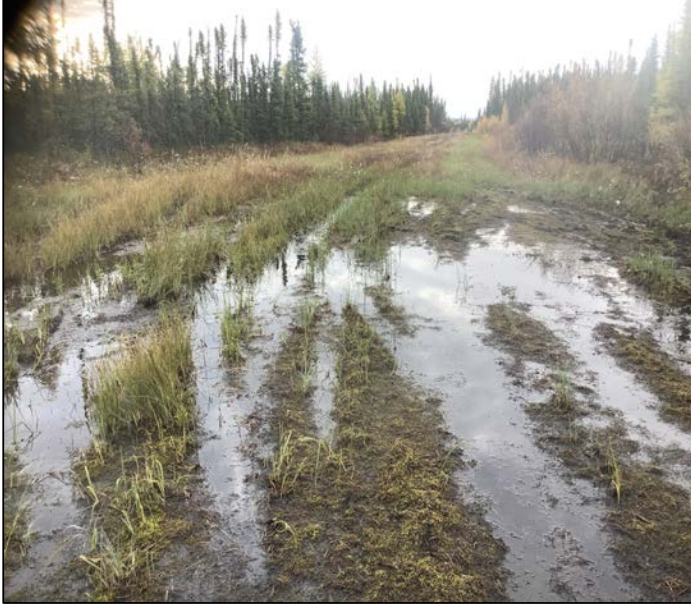
Photo 1. Facing south on existing winter road
