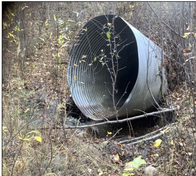
Photo 2. Facing left downstream bank towards inlet
