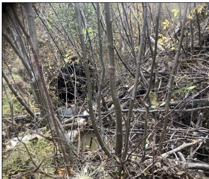
Photo 3. Facing downstream towards culvert inlet
