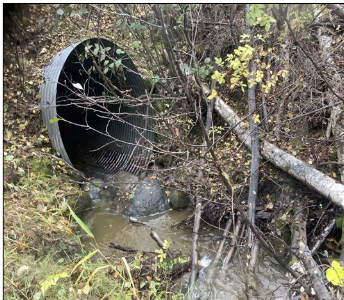
Photo 4. Facing downstream towards culvert inlet
