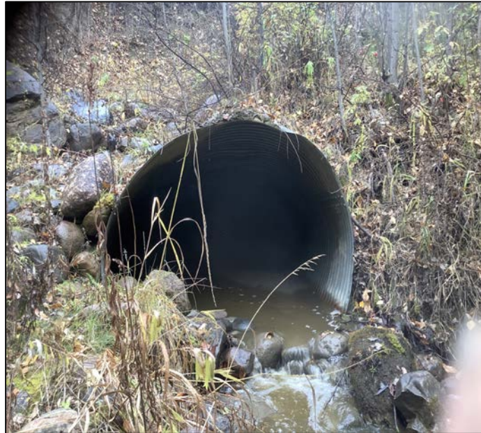
Photo 2. Facing outlet of culvert
