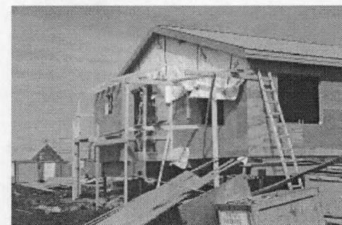
Exterior of a housing unit nearing completion.
